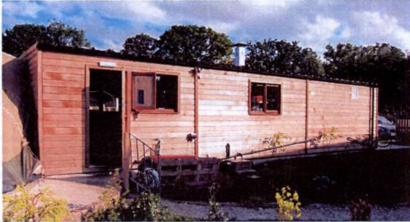
Photograph 1 The Camp Kitchen from the north west
