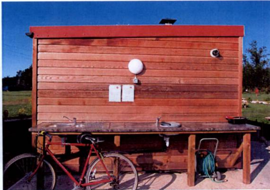
Photograph 3 the south west elevation showing the 2 sinks available for the use of camping visitors
