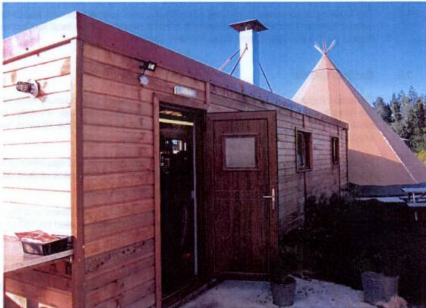
Photograph 2 The Camp Kitchen from the south showing its relationship to the Canteen Tent or Café
